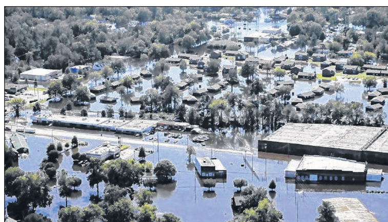
This photo from 2016 shows the flooding in Lumberton caused by Hurricane Matthew.
