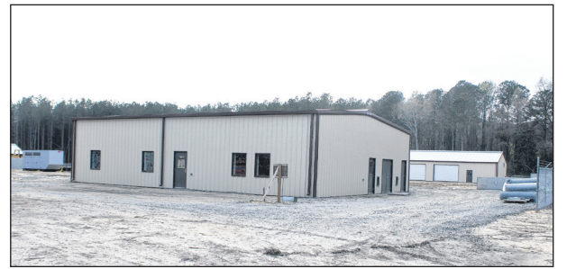
Chris Stiles | The Robesonian A structure has been built at the site of the new Wastewater Treatment Plant in St. Pauls.
